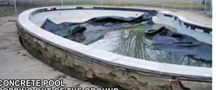
CONCRETE POOL POPPING OUT OF THE GROUND DUE TO FAULTY HYDROSTATIC VALVES
